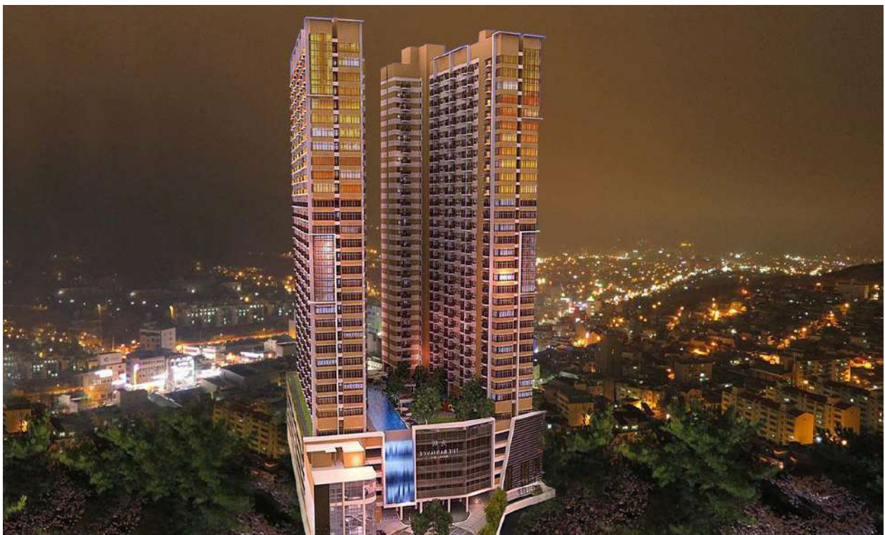
THE RADIANCE MANILA BAY – ROXAS BLVD., PASAY CITY
