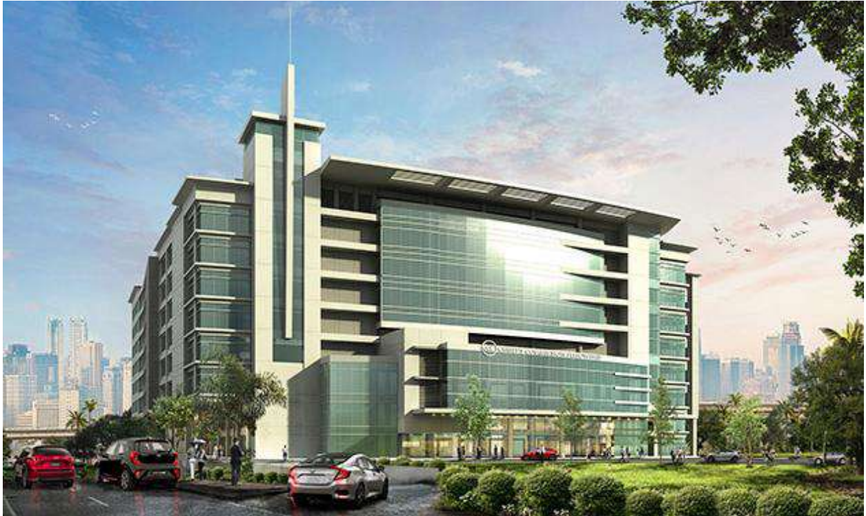
CCF 20 STOREY BUILDING – PASIG CITY
